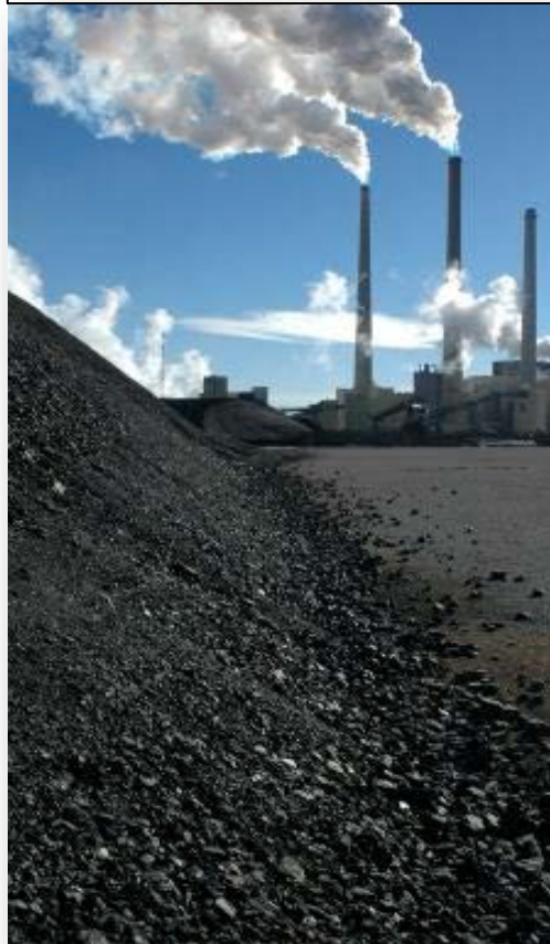
Air Pollution Control
